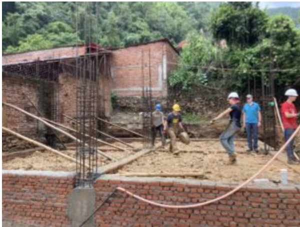
Filling the foundation.
