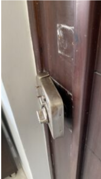
Our bent, non-functioning lock
