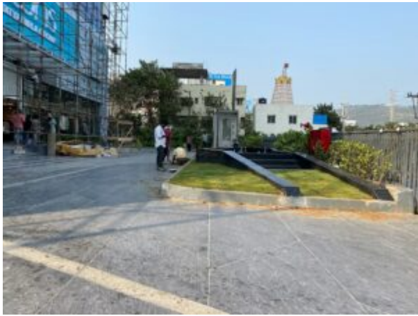
Laying sod at Lansum Square entrance
